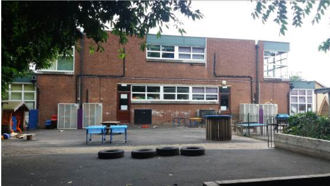
Remaining school building to be demolished
